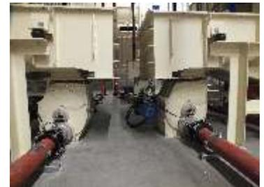
Manifold arrangement allowing any of the blowers to be selected to feed any of the conveying routes. Each line is fitted with a pinch valve near its destination to permit line isolation and prevent material back flow from the mixer. Product mixing is via an existing trough blender which was modified to incorporate a radial gate discharge system and a top mounted reverse jet filter unit.
